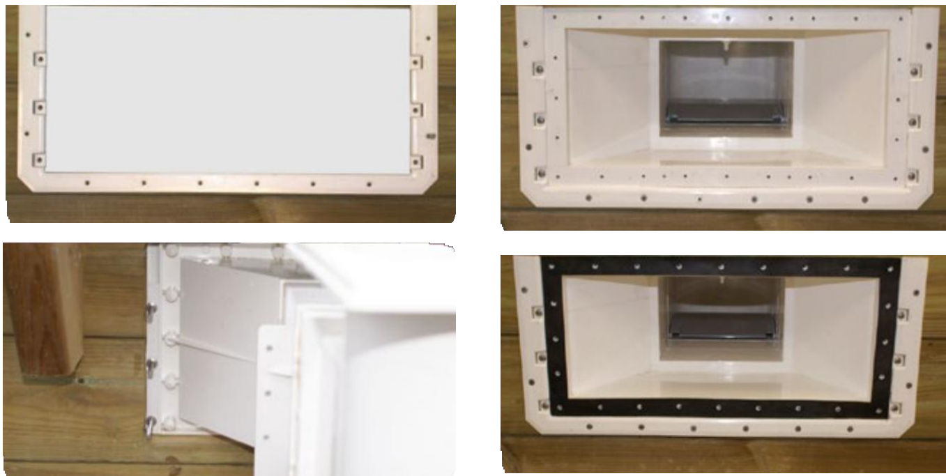
Figure 21 – Montage du skimmer
